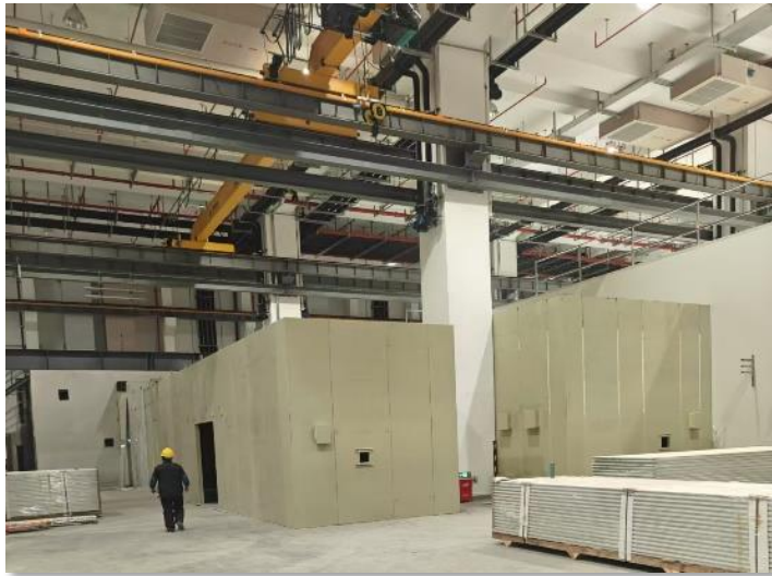
Constant temperature shed completed
