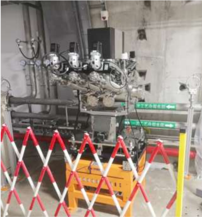
Solid Attenuator @ 1134m Finished Installation
