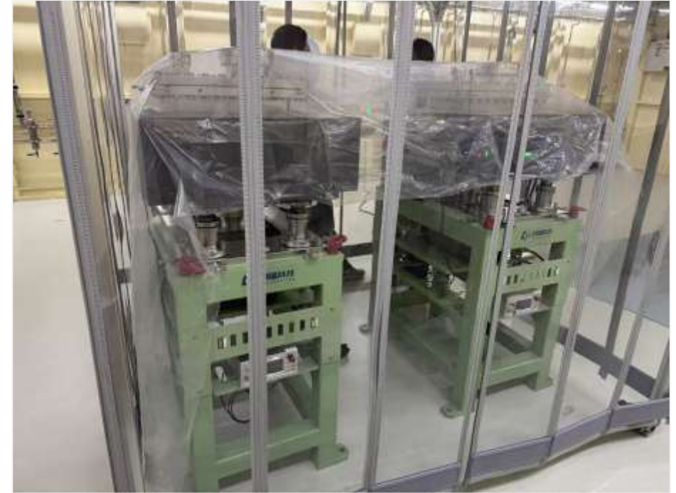
Ref. Laser @ 1141.8m & 1170m Ready for Installation
